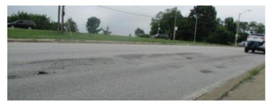
PHOTO 4-6: TYPICAL HANOVER STREET PAVEMENT RUTTING
